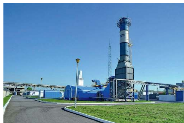
PHOTO 3. Test bench for gas turbine engines AL-31ST
