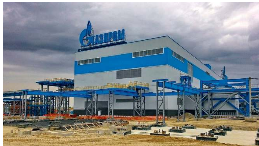
PHOTO 6. Grozny TPP under construction
